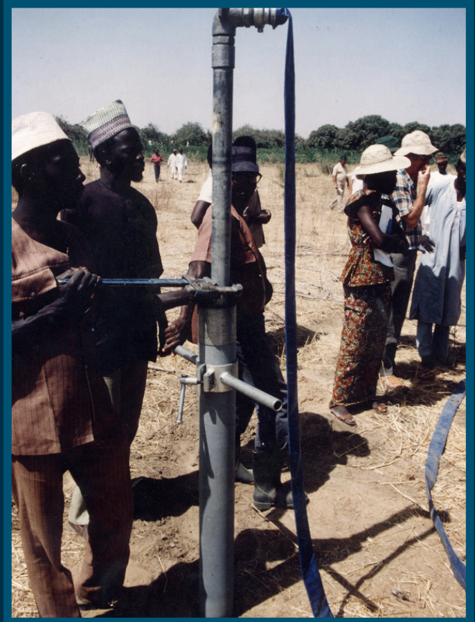
Manual dilling, Northern Nigeria
