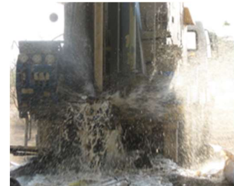
Drilling into a water bearing fracture in Kenya
