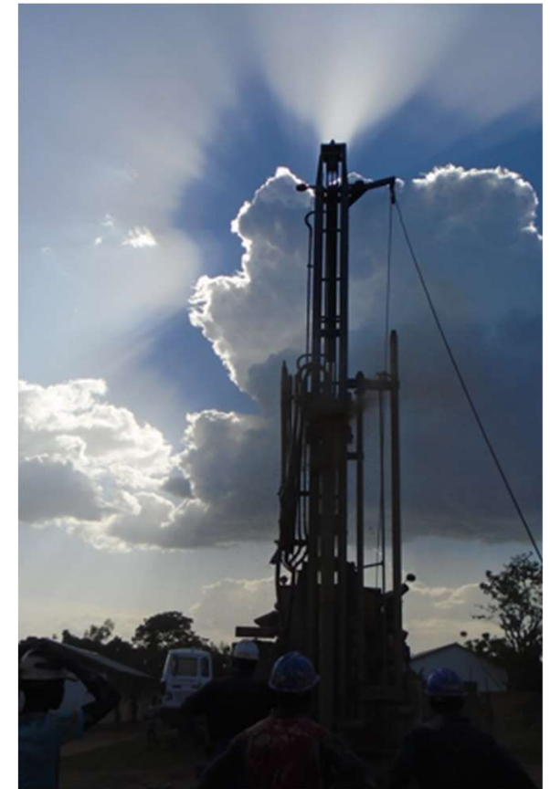
GWR successfully supported MSF-OCP with the drilling of a production borehole for Paolo Hospital, CAR
