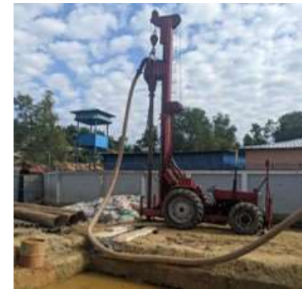
GWR drilling a production well in Teknaf, Cox's Bazar, Bangladesh
