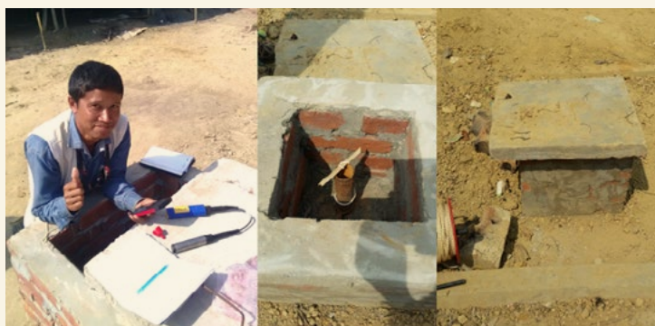
Figure 48: Installation and operation of in situ groundwater level loggers at an MSF-OCA monitoring borehole, including staff training, secure housing of monitoring equipment, and routine data download procedures. (GWR)
