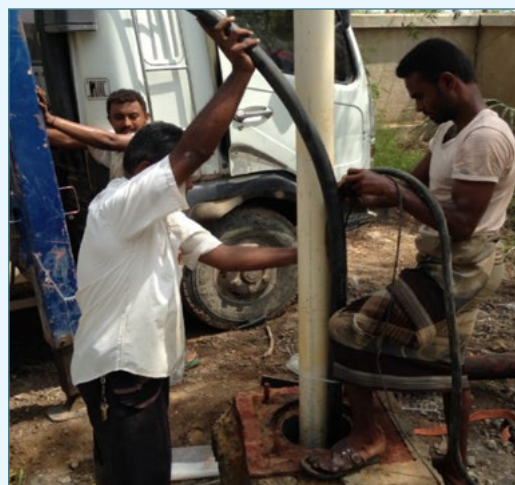
Figure 31: Dip tube installation in Al Mokha well field, Yemen. (GWR)
